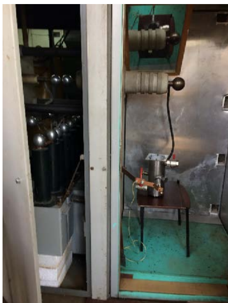
Figure 1 – Installation for generating high-voltage discharges in water
